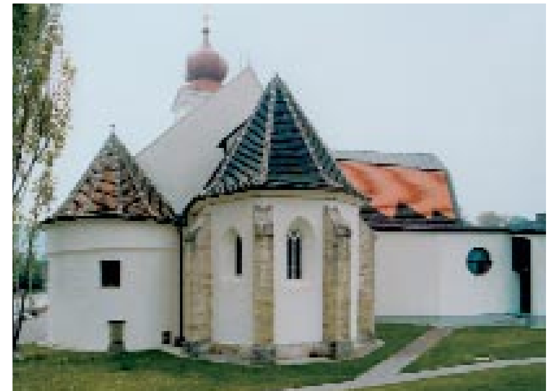
1, 2. Floor plans of the church before and after conversion. 3. View from the south-west. 4. View from the north-east.
