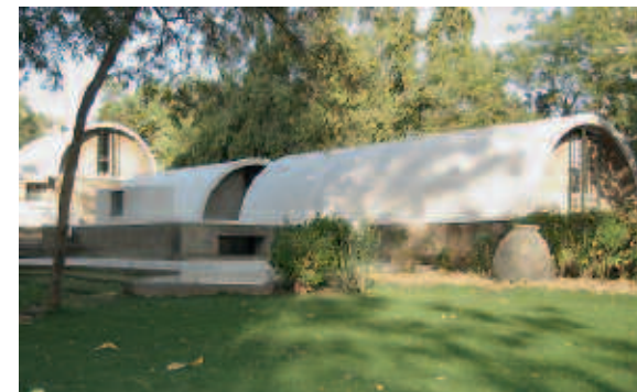
Figure 8.26 White, glossy roof: solar absorption: 0.2 Exterior wall color light brown, solar absorption: 0.6 (Sangath, Vastu-Shilpa Foundation, Ahmedabad)
