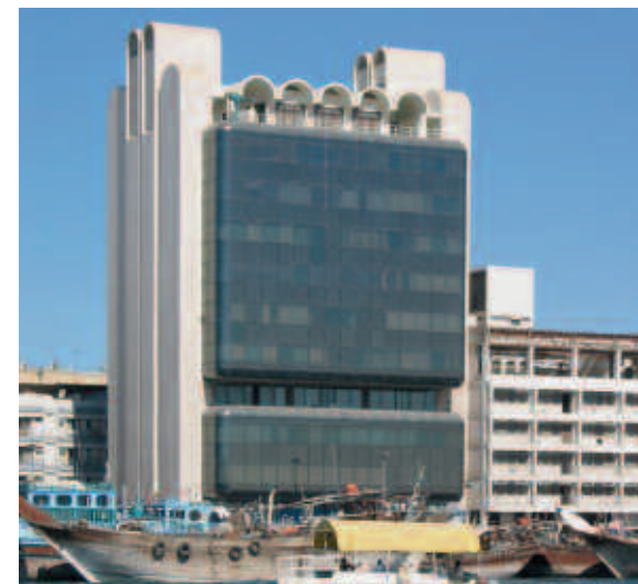
Figure 8.27 Dark glass façade: Solar absorption: 0.75 Light exterior wall colors, solar absorption: 0.3 – 0.4 (office building in Dubai, UAE)
