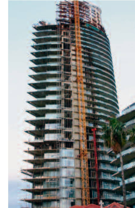
Figure 8.2 Reinforced concrete frame construction in the Middle East; Beirut (Lebanon) 2006
