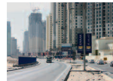
Figure 8.3 and 8.4 Reinforced concrete frame construction in the Middle East; construction boom in Dubai (UAE) 2006
