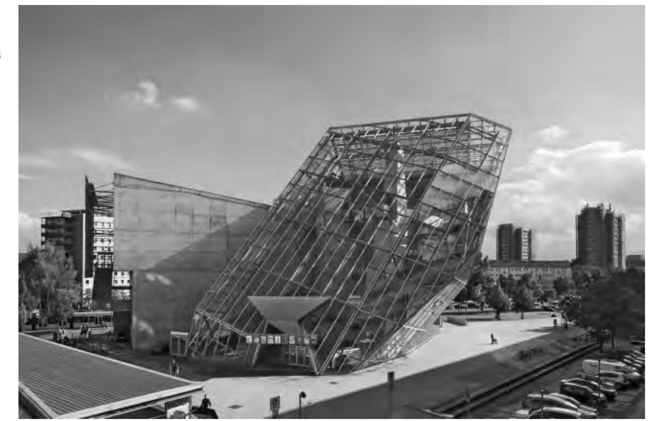
entrance. Outside it is protected by an inclined awning, directly fixed to the main frame and, like the Cloud, clad in steel sheets.
