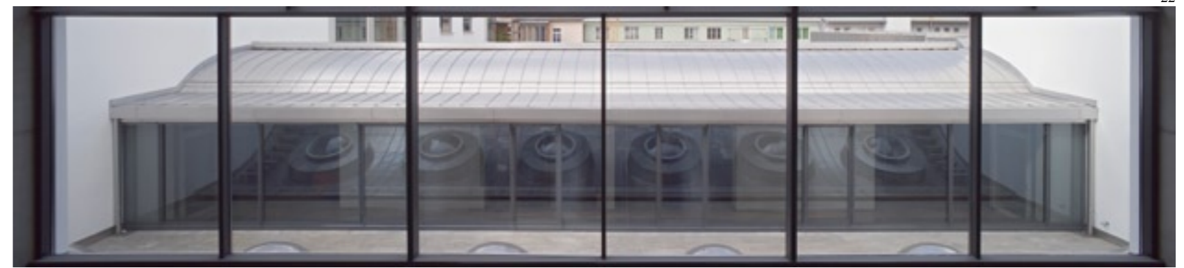
20 Customer service centre, hall on the 4th floor. 21 Undulating roof with Nordkette range. 22 3rd floor lateral section.
